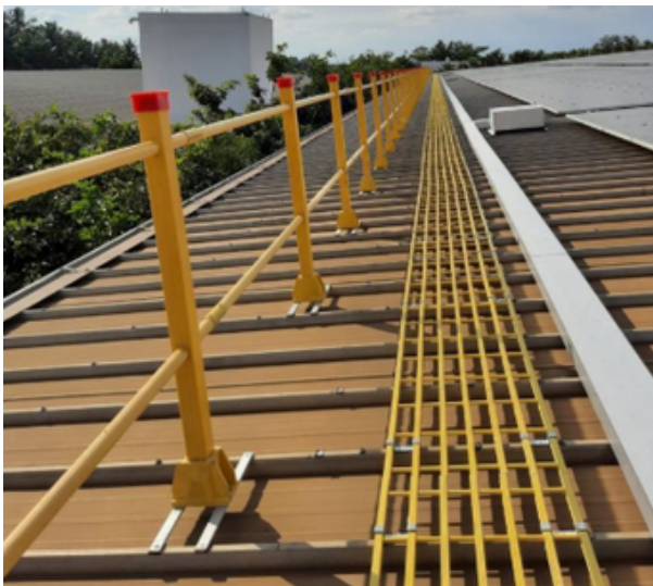
Solar Rooftop Handrail
