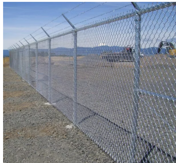
Switchyard Mesh wall material
